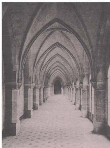
The Large Cloister
